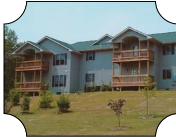
Woodstone at Massanutten McGaheysville, Virginia
